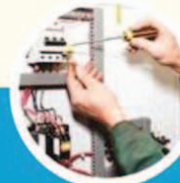
Electric and grinding Work
